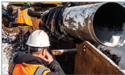
DI pipe can be assembled in nearly all weather conditions.
