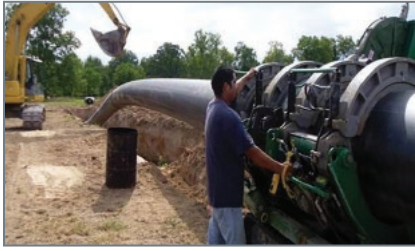
HDPE must be welded together with special machinery.
