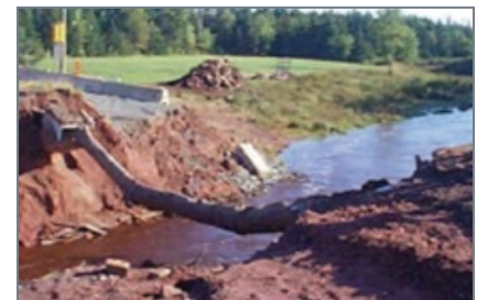
Resilience of DI pipe to trench loss
