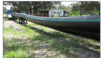
HDPE must be assembled above ground in optimal weather conditions.
