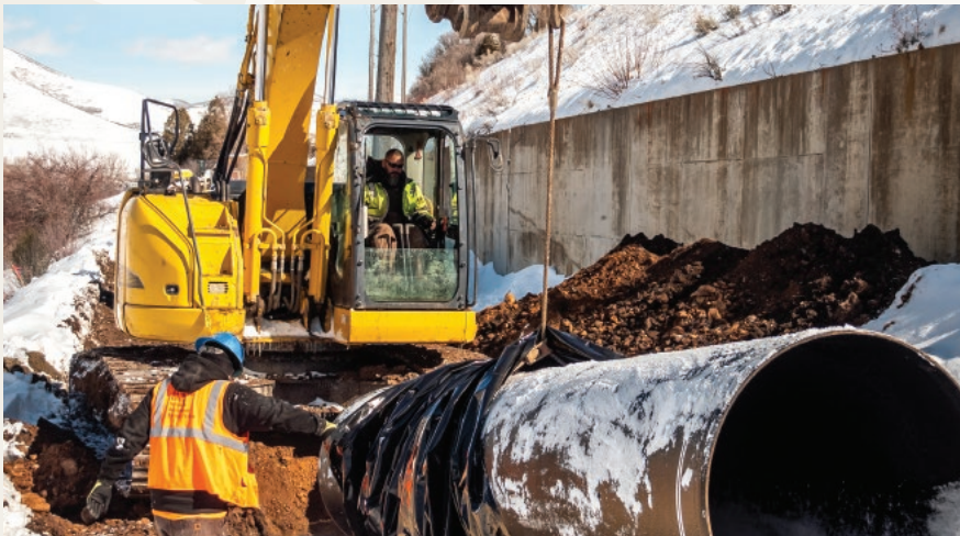
Ductile iron pipe being installed without concerns in subfreezing snowy conditions
